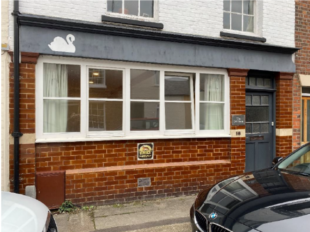
Good example of shopfront to residential conversion. This residence was formerly a pub and has retained its traditional fascia and tiled stallriser. This façade provides sufficient privacy while retaining the shopfronts original windows (Source: RBC Planning).
