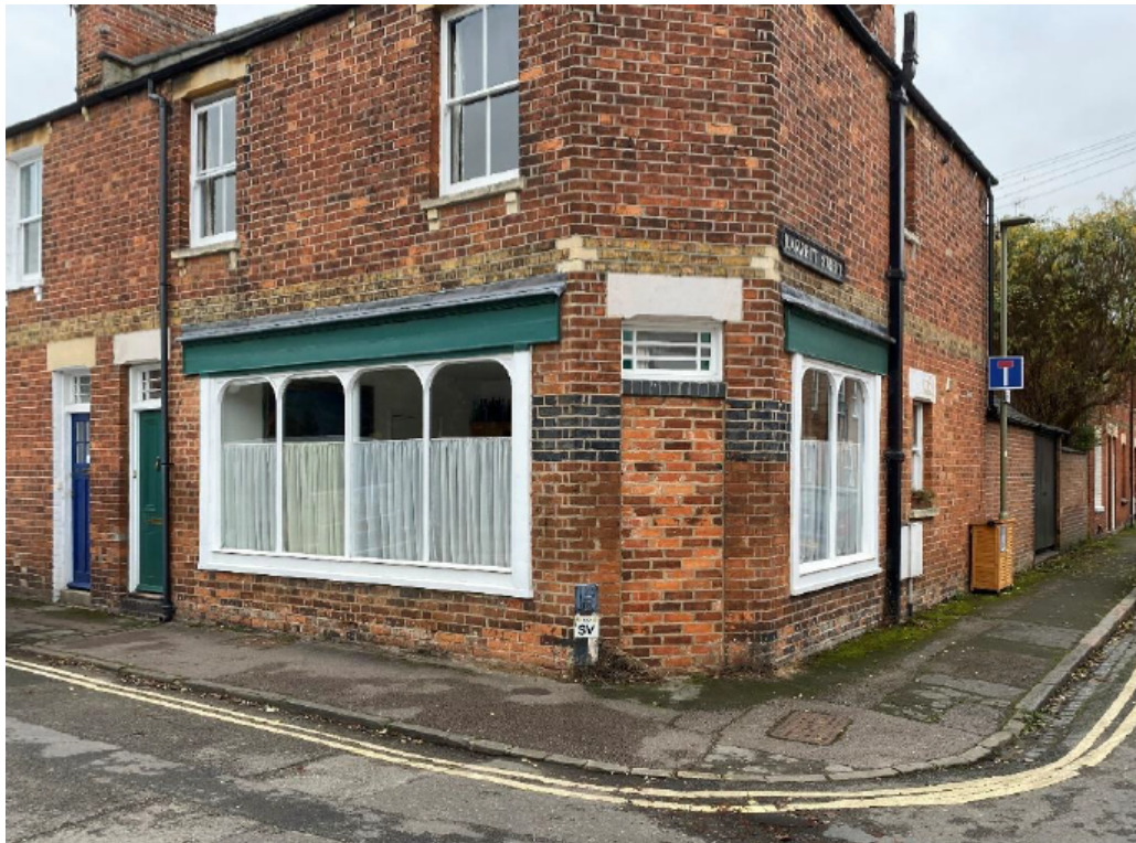
Good example of a shopfront to residential conversion. It retains the fascia and shopfront windows, as well as the distinct glazing above the former shopfront's doorway on the corner. (Source: RBC Planning).
