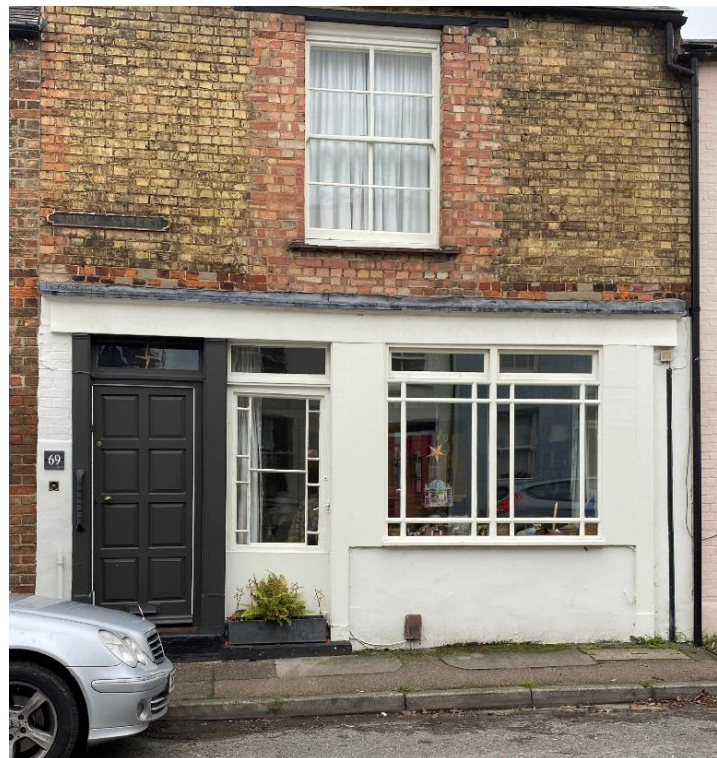
Good example of a shopfront to residential conversion. This conversion retains the shopfront's stallriser and display windows. (Source: RBC Planning).
